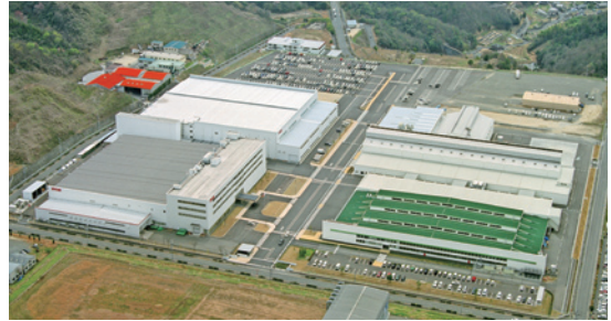
Hiroshima East Plant (the die casting facilities are on the right)
