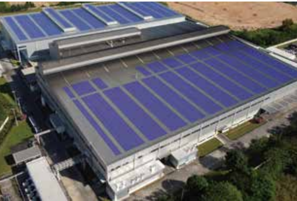
Solar panels installed at Ryobi Die Casting (Thailand) Co., Ltd. (image of completed installation)
