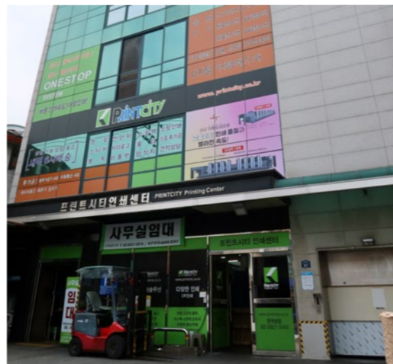
10-story head office building
